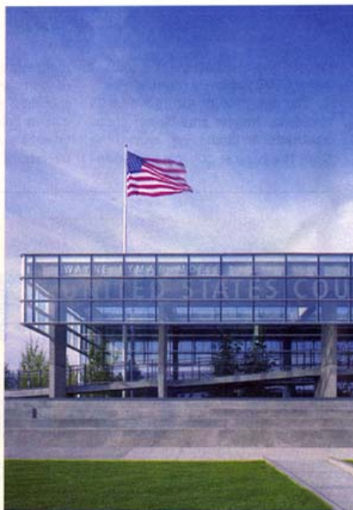
THE ENTRY: The outer staircase evokes the Supreme Court building while also impeding car-bomb attacks.
